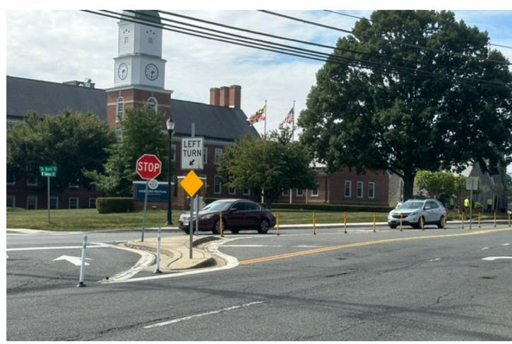
Flex posts are used to close the left turn onto E Gordon St, which simplifies the intersection (Source: Laura Bianca-Pruett, Town of Bel Air)
